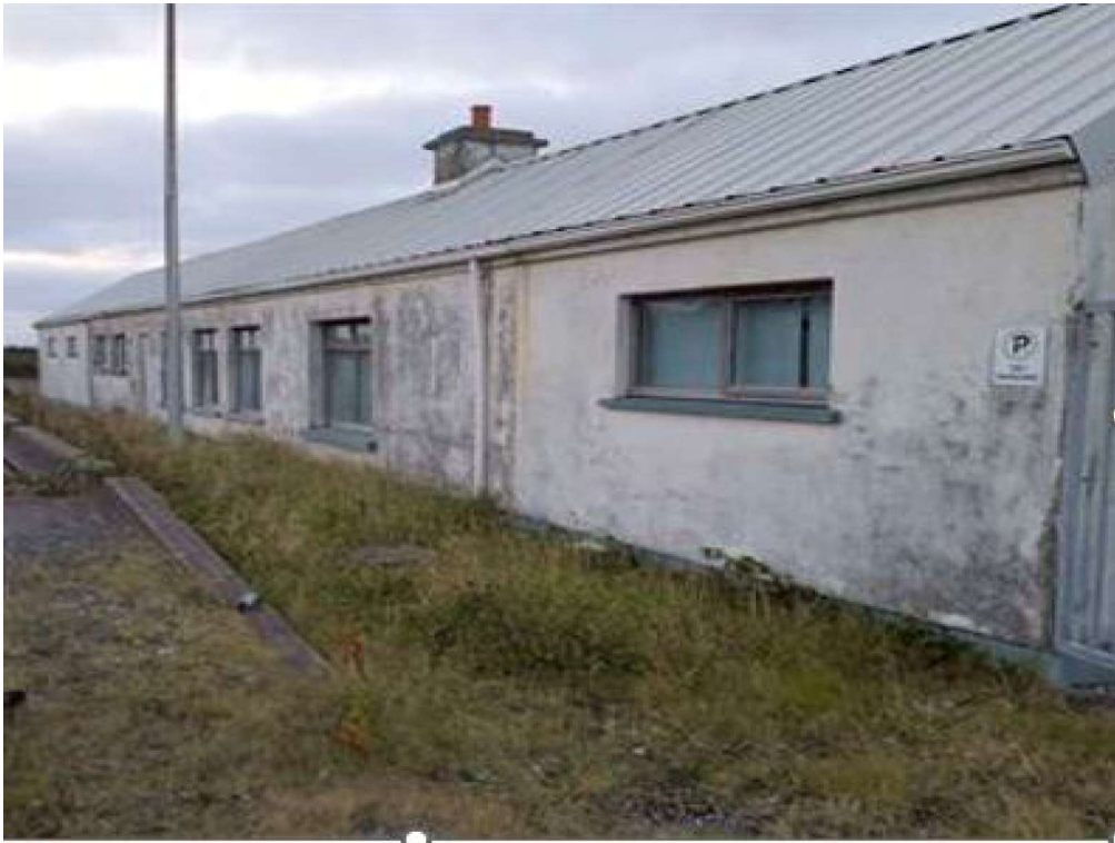
Plate 7: Southwest face of old office building (F.4) (54143322, -9.895129)
