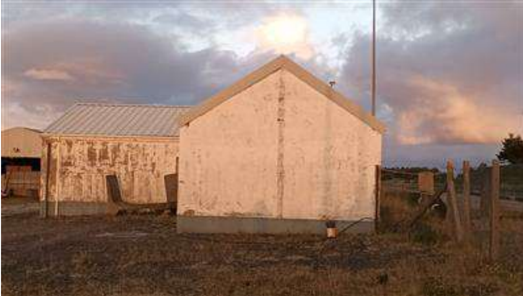
Plate 1: North face of office building (F.5) (54.143658, -9.895703)
