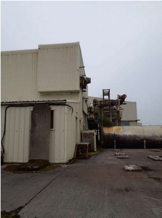
Plate 3: North side of old metal factory (F.3) (54.143657, -9.893473)
