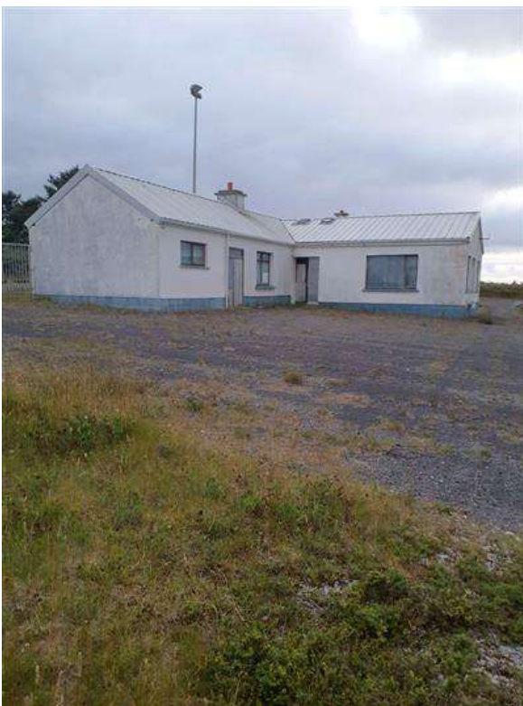
Plate 6: Southeast side of old office building (F.2) (54.143373, -9.894731)
